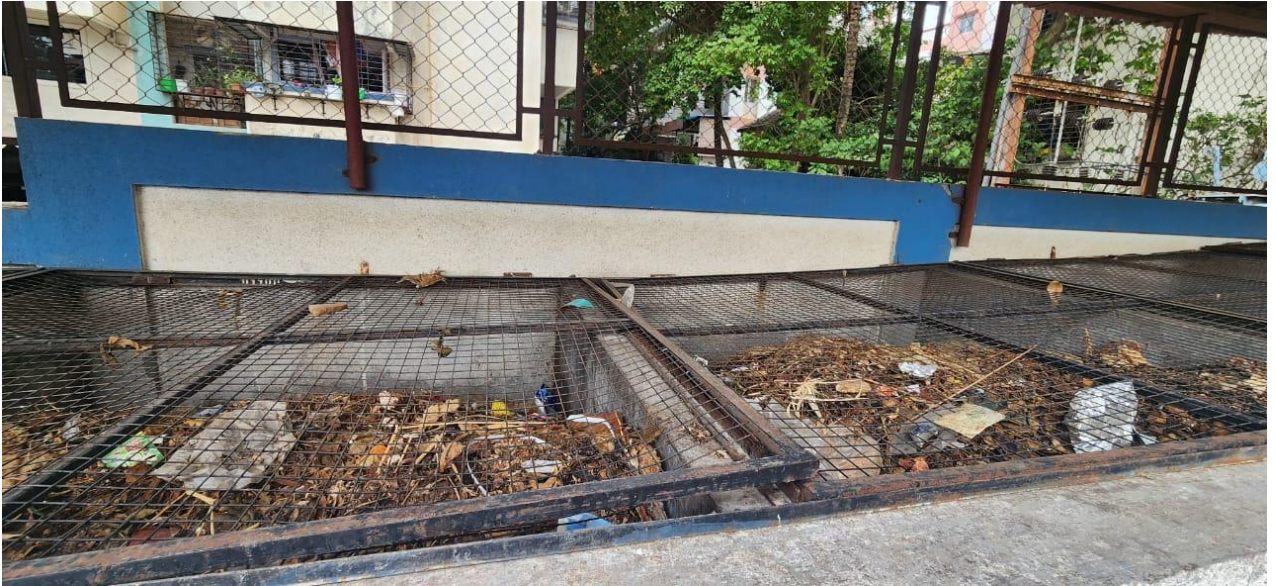
7 Pits – for treatment of wet waste
